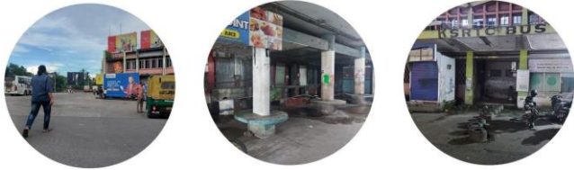
Figure 8,9,10: Condition of KSRTC bus stand Source: Author
